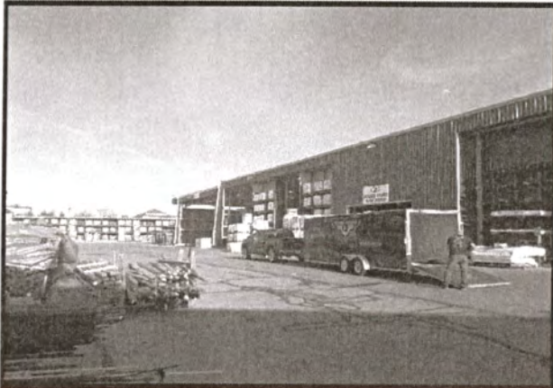
Northeast Section of Building (2014 Addition)
