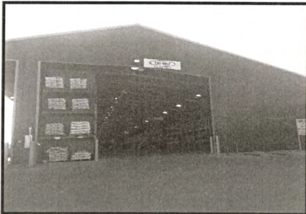
Lumber Shed - East Elevation (Exit)
