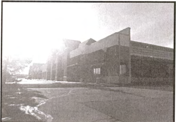
View of South Elevation
