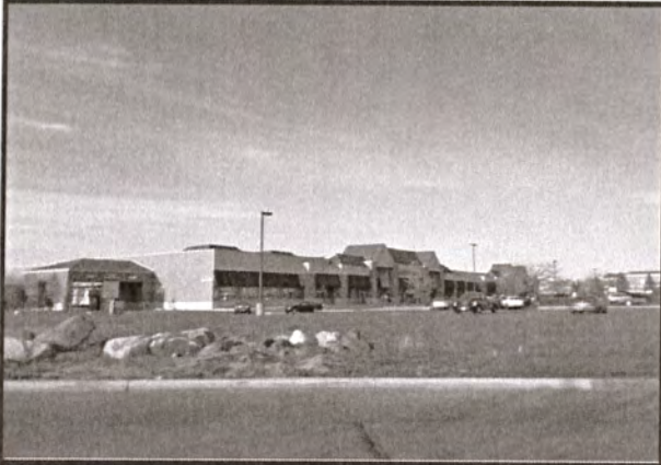
West and South Elevations - Facing Northeast
