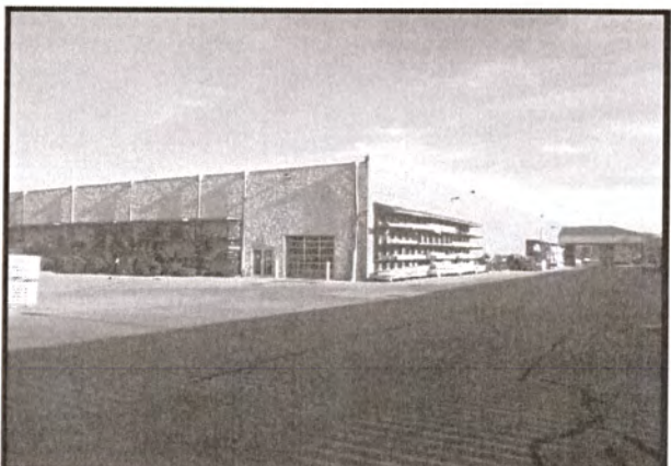
North and West Elevations - Facing Southeast
