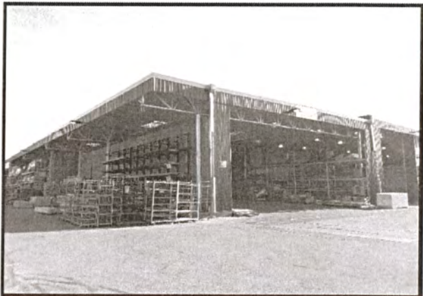
Northeast Section of Building (2014 Addition)
