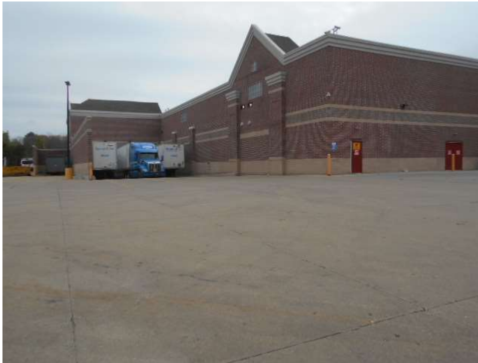
Exterior Truck Dock Doors
