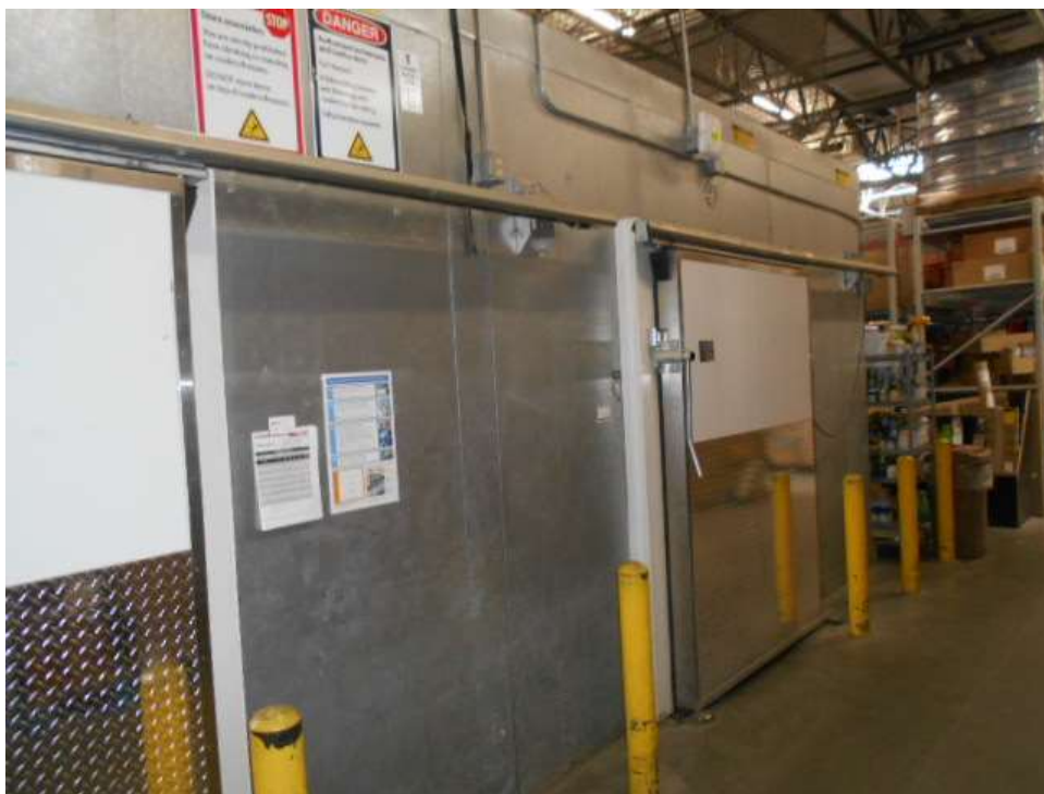
Backroom Storage Area
