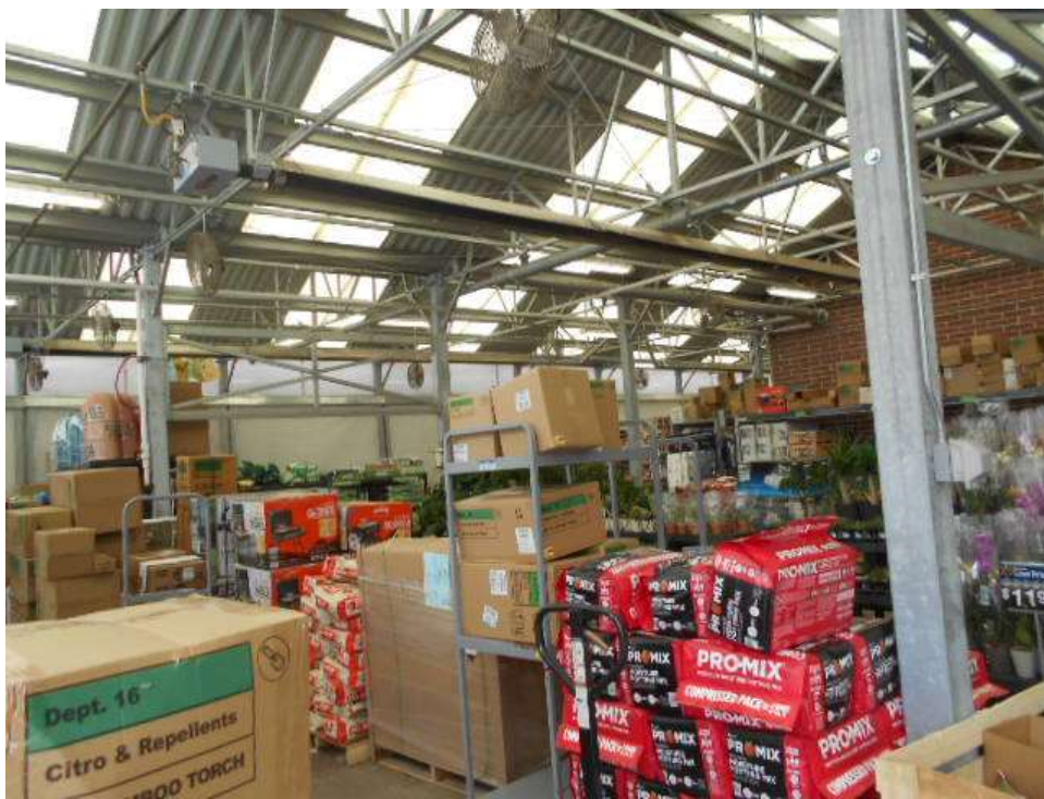
Exterior Sales/Storage Canopy Area
