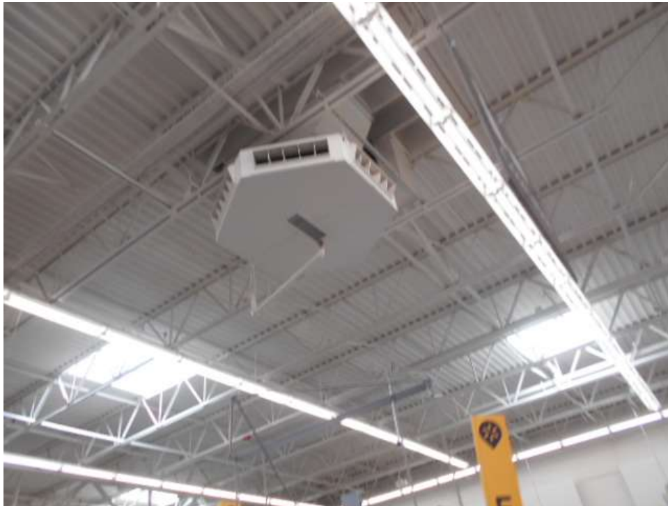
Sales Floor Ceiling
