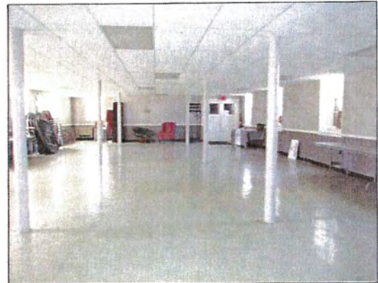
28. Basement area main church.
