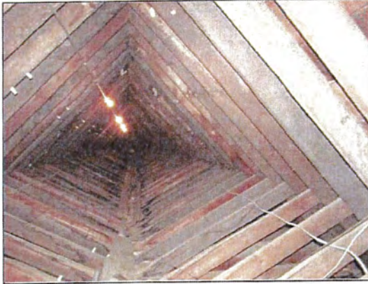
19. Scissor trusses in the church attic.
