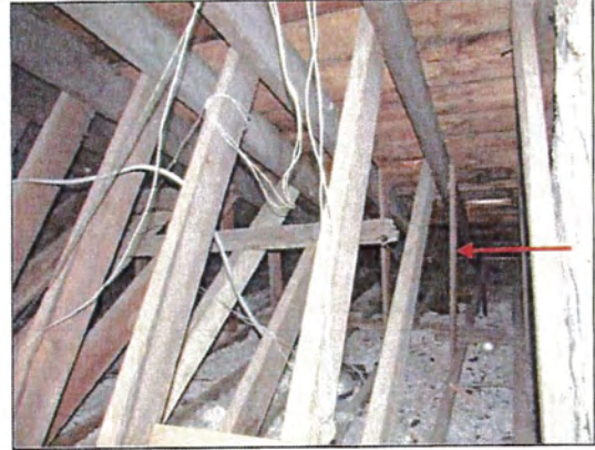
20. View into attic perimeter. Note vertical plater supports.
