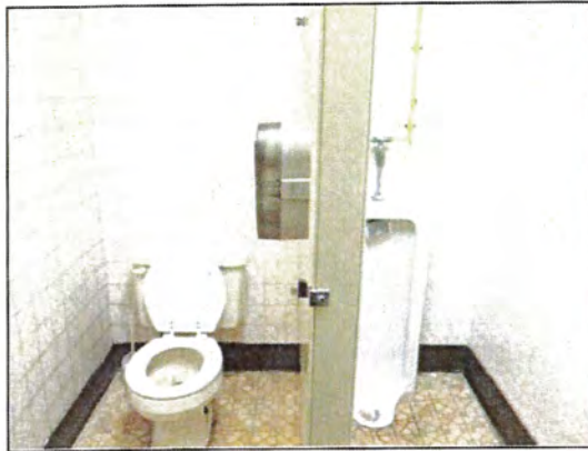
33. Existing men's room.
