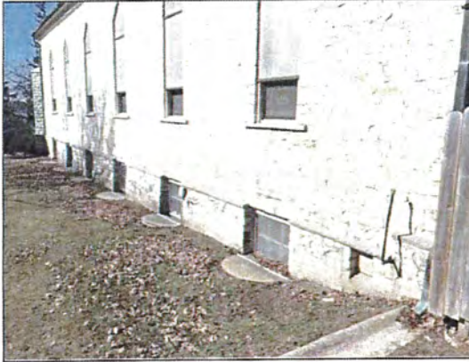
1. East elevation of main church building.
