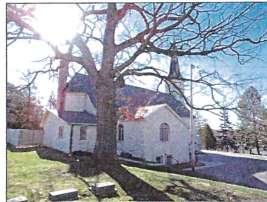
4. North elevation view from the west.
