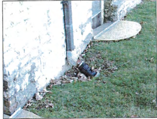
8. West elevation of church building.
