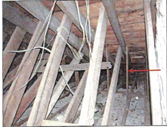
32. View into attic perimeter. Note vertical plater supports.
