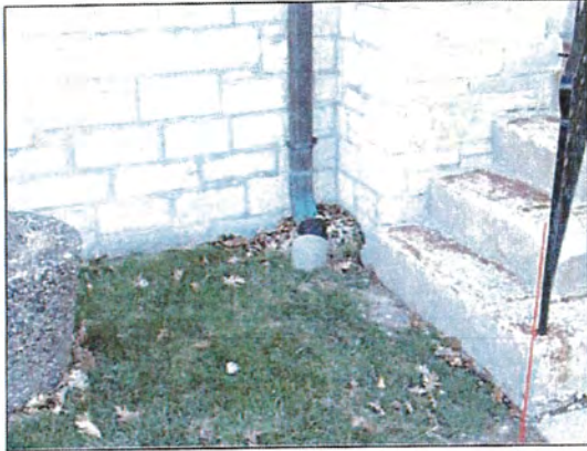
7. At annex stair entrance.
