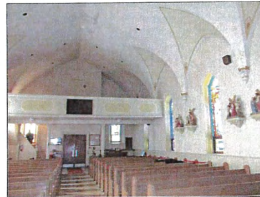
16. Interior view looking south.
