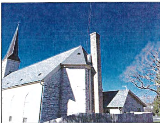
5. North elevation view from the east.
