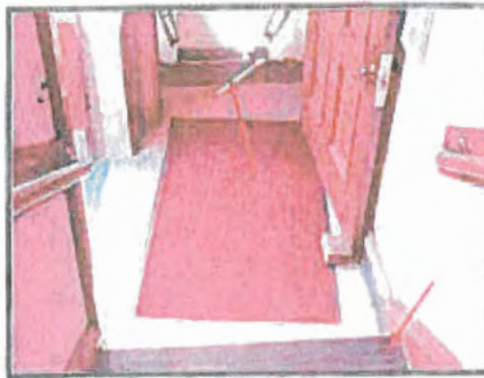
23. Annex entry is below floor line of church (foreground) with stairs leading to basement.
