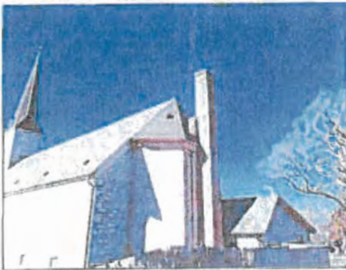
5. North elevation view from the east.
