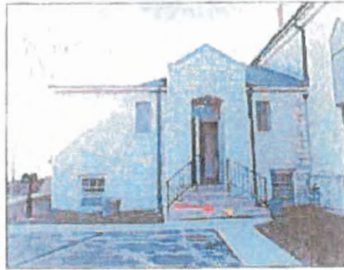
14. Annex entrance, south elevation. Note the trip hazard painted yellow.
