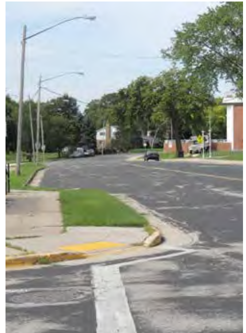
A recent photo of Garfield Drive reveals the ample width available for adding angled parking as proposed below
