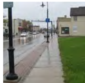
Existing terrace treatment
