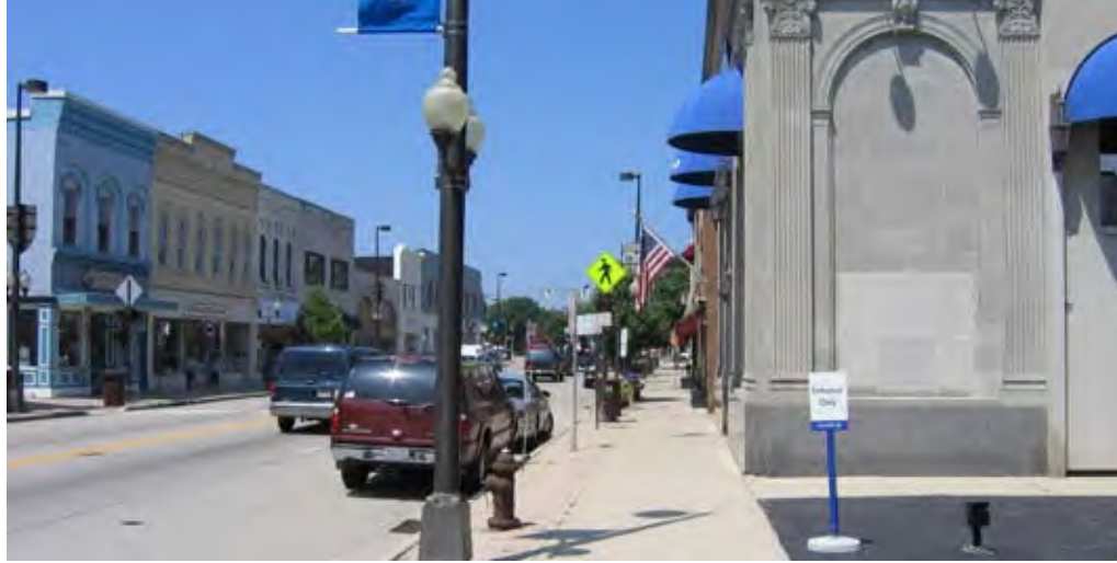
Streetscape prior to improvements
