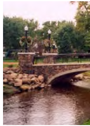
Mill Pond pedestrian bridge
