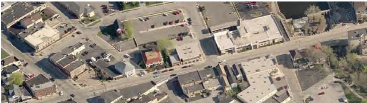
Village Centre Aerial
