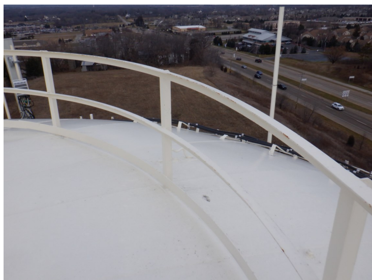
27) The center handrail is in good condition.
