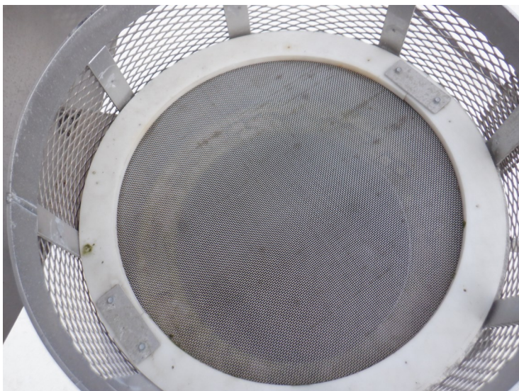
36) The interior screen is in good condition.
