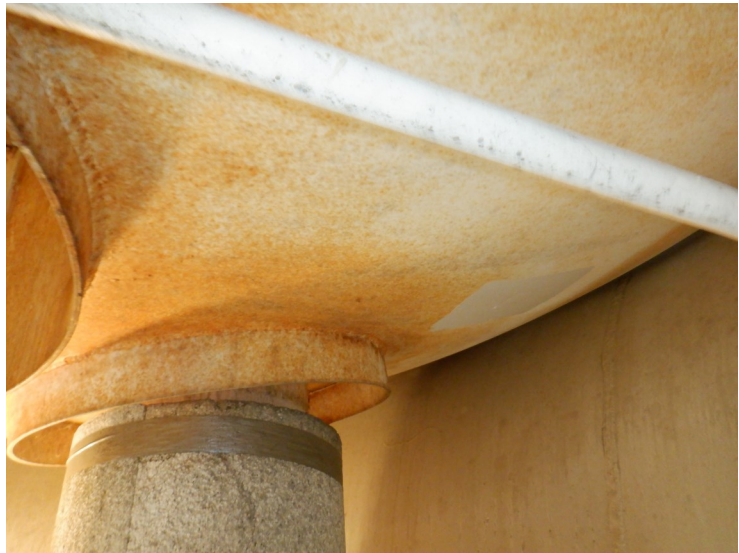
44) Extensive rust bleedthrough on the bowl.
