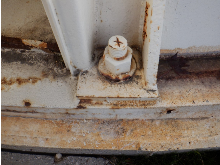
1) The foundation, grout, and anchor bolts are in good condition.
