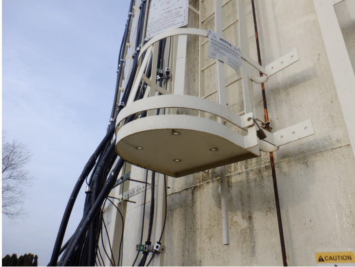
10) The sidewall ladder vandal guard is in good condition.
