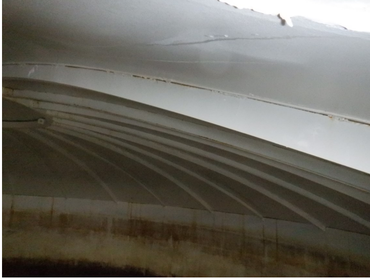
43) The roof stiffeners are in good condition.
