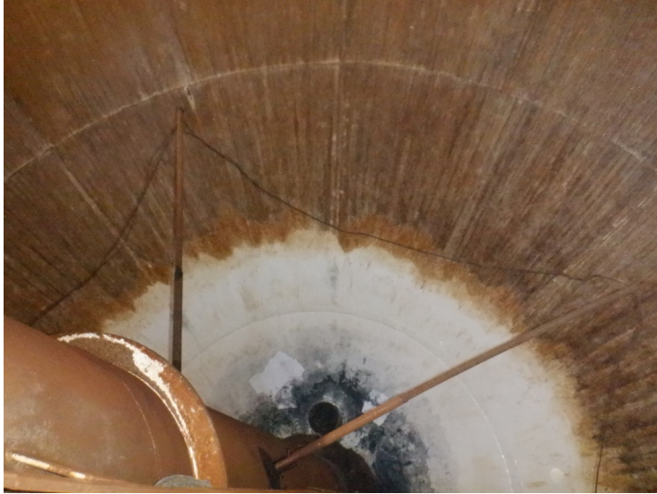
58) The cathodic protection system appears to be in good condition.
