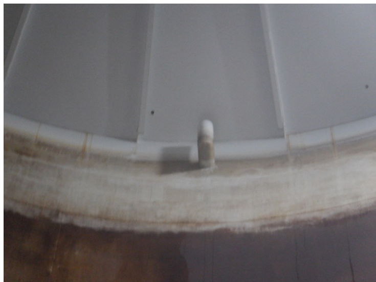
45) The overflow elbow is in good condition.
