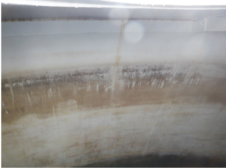
46) The coating on the sidewall is in good condition overall.
