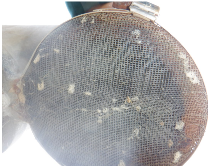
5) The roof vent screen is intact.
