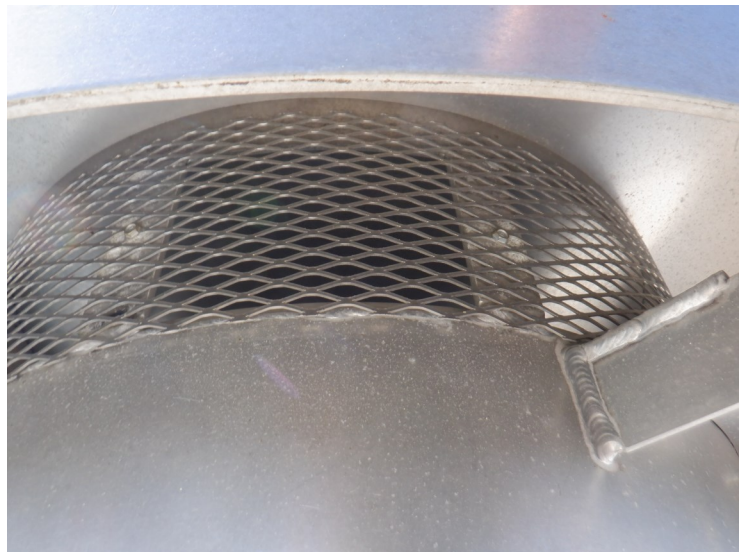
23) The vertical roof vent screen is in good condition.
