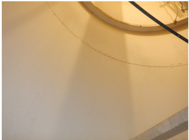
35) The dry riser coating is in good condition overall.
