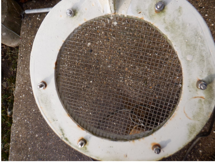
7) The screen is in good condition.
