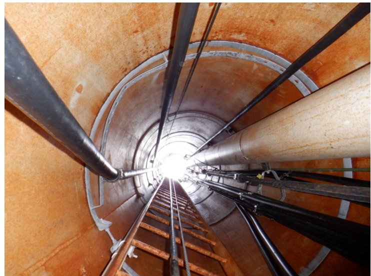
50) The access tube ladder is in good condition. The ladder is equipped with a fall prevention device.
