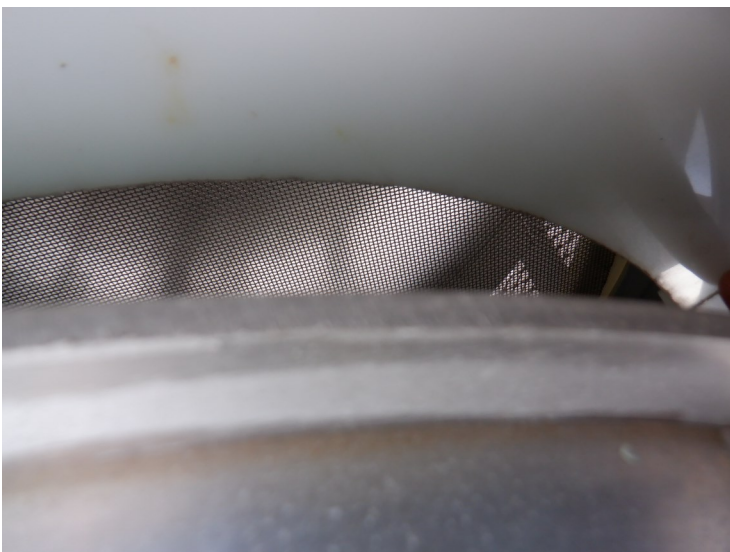
24) The interior roof vent screen is intact with no gaps.
