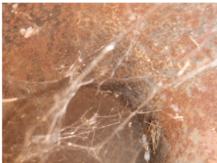
3) The screen at the overflow discharge is intact with no gaps or holes.
