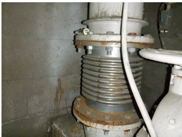
69) The bellows type expansion joint on the fill/draw pipe is in good condition.
