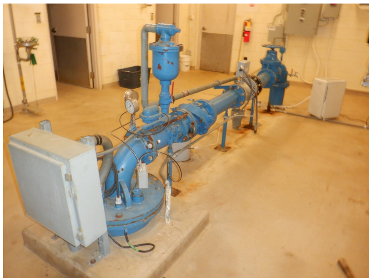
69) Coating on the piping in the building is in fair condition.
