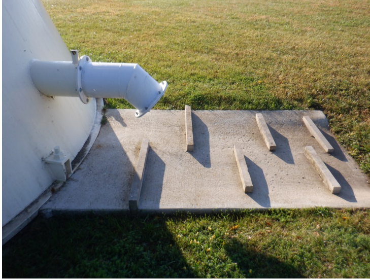
4) The overflow pipe discharges to a concrete splash pad.
