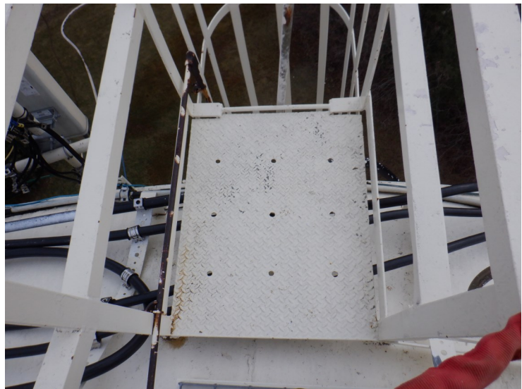
23) The step-off platform is in good condition.
