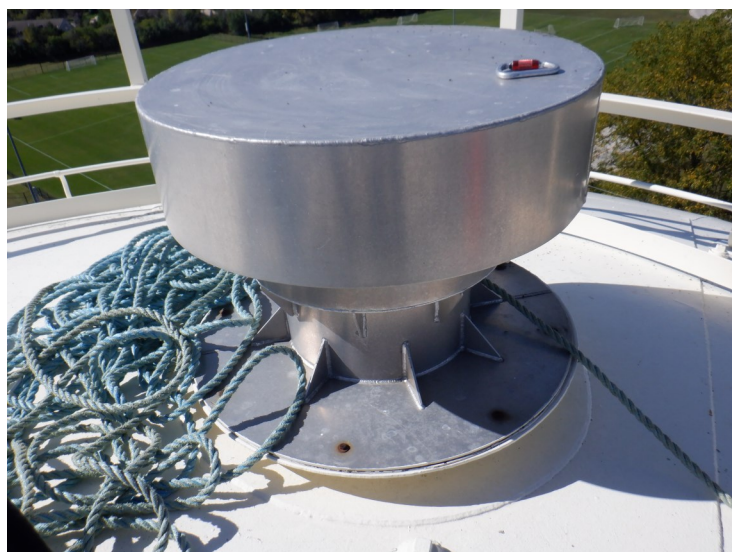
21) The roof vent is in good condition.
