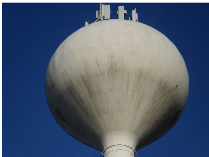
18) The sidewall coating is in good condition overall.
