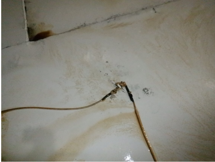
58) There are cathodic clips on the floor.
