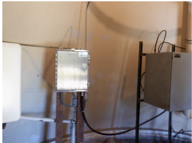
26) The dry interior basebell coating is in good condition overall with no significant deterioration.
