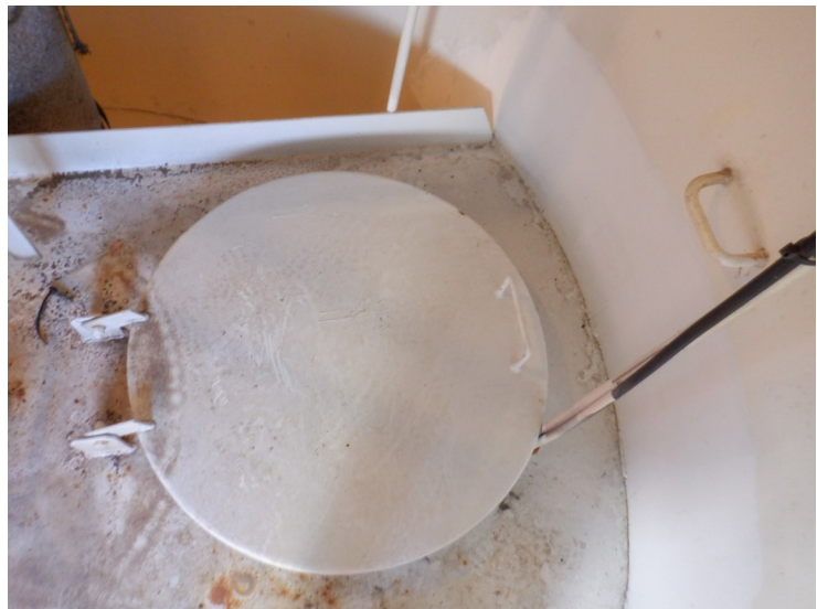
38) The ladder opening at the top platform is equipped with a hinged cover.
