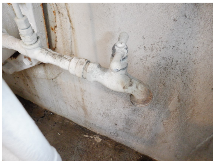
63) The sample tap is in good condition but has a threaded end.
