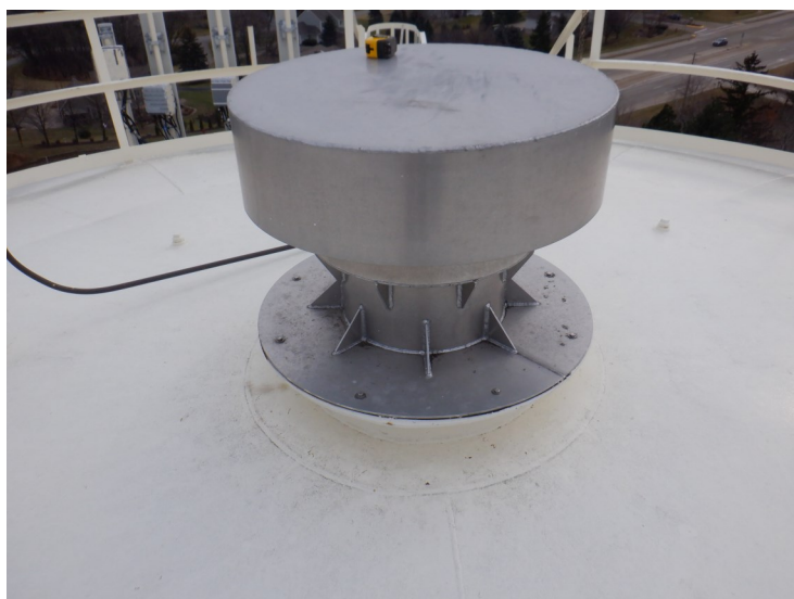
33) The roof vent is in good condition.
