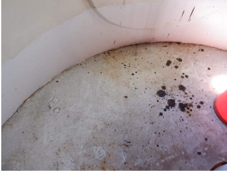
40) Coating on the top platform is in good condition overall.
