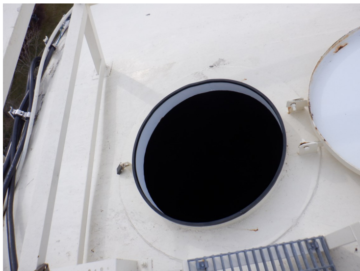
39) A roof hatch gasket was installed by the inspection crew.
