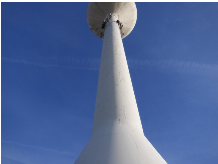
12) The riser coating is in good condition overall.
