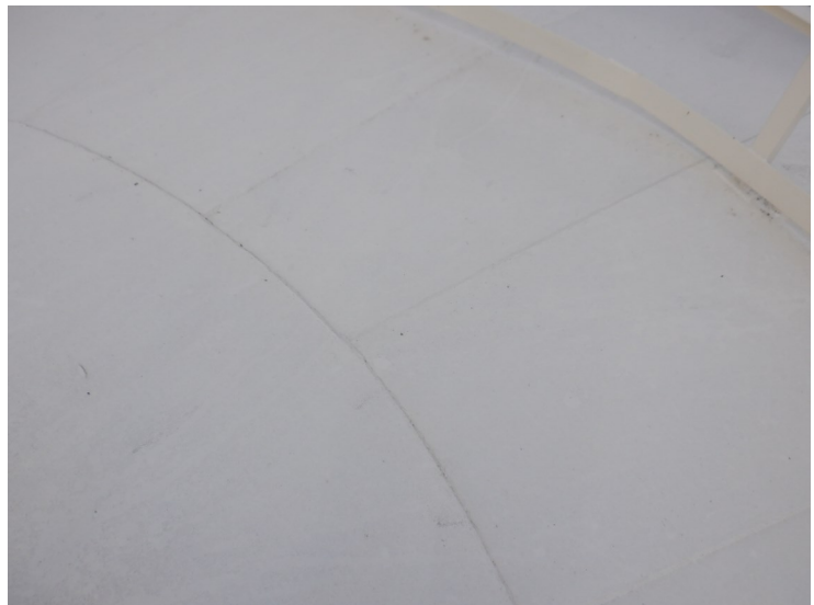
20) The coating on the roof is in good condition overall.
