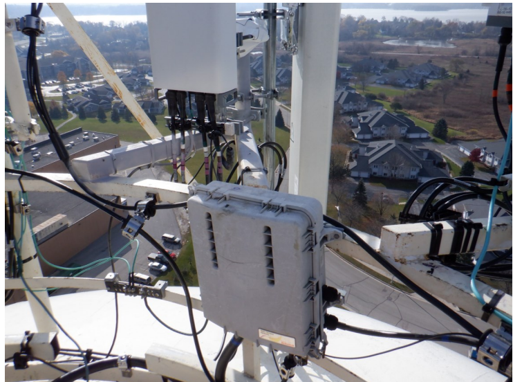
23) The roof handrail is in good condition. There are antennas attached to the roof handrail. There is not a painter's railing on the roof
