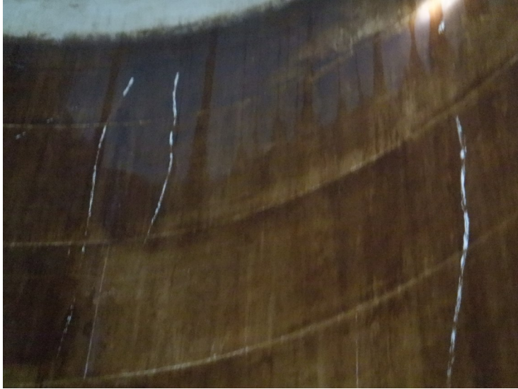
49) The scratches could be a sign of ice movement.
