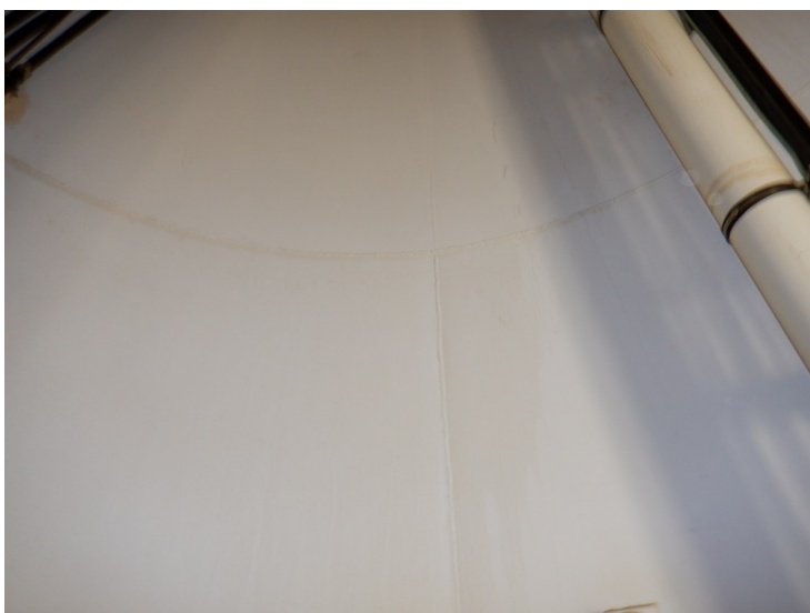
30) The dry interior basebell coating is in good condition overall.
