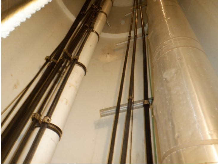
40) The fill/draw pipe insulation and aluminum cover are in good condition.
