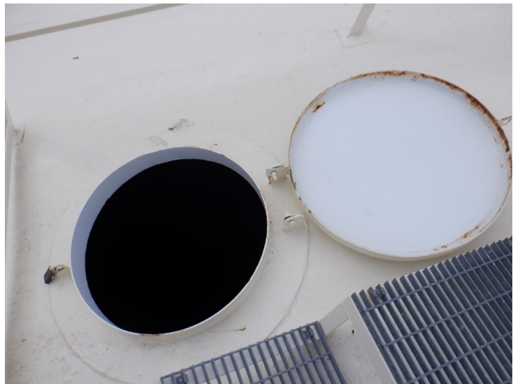
38) The roof hatch is in good condition.
