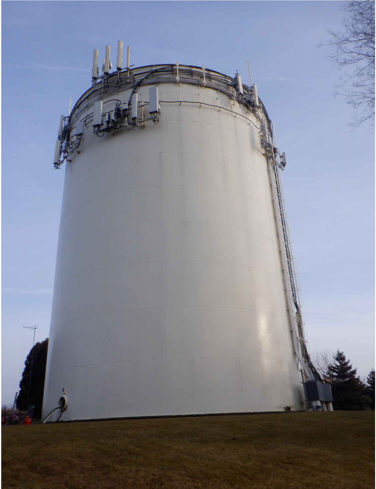
1,000,000 gallon standpipe (Sunnyridge) located in the Village of Pewaukee, Wisconsin.
