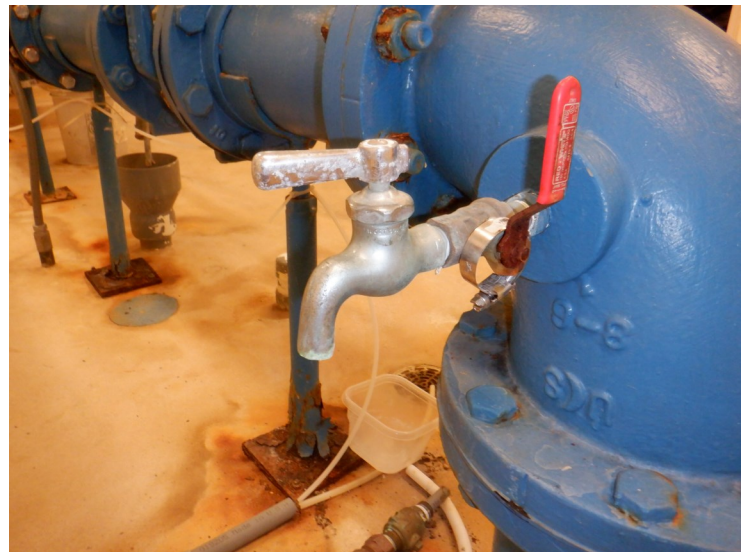
71) The sample tap in the building is in good condition.
