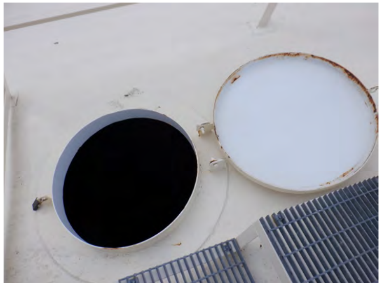
38) The roof hatch is in good condition.
