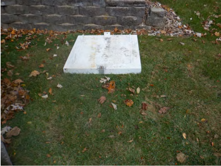
7) The roof hatch covers are in good condition with some coating erosion.
