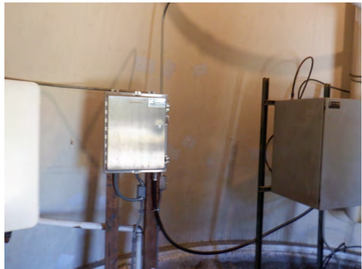
26) The dry interior basebell coating is in good condition overall with no significant deterioration.
