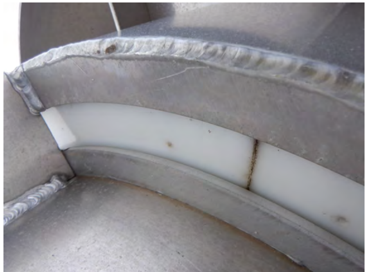
35) The pressure plate is in good condition.
