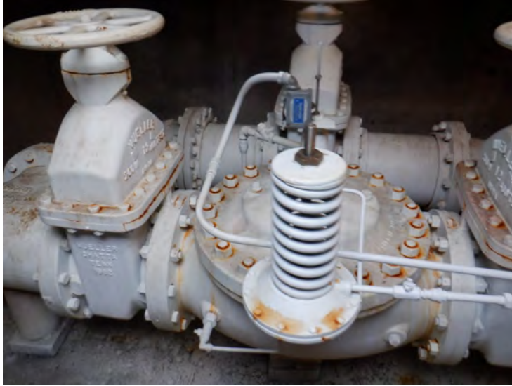
64) The coating on the piping is in good condition overall.
