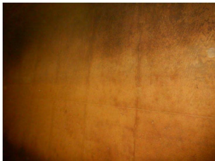
12) The concrete sidewalls are in good condition with no significant deterioration.
