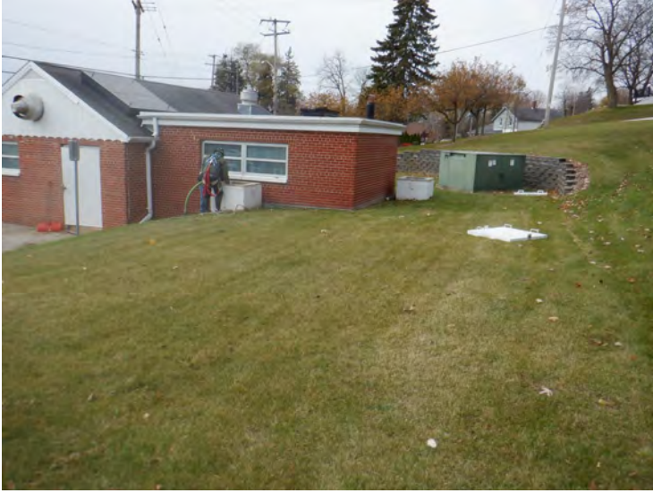
1) 125,000 gallon underground concrete water storage reservoir (Well 2) owned by the Village of Pewaukee, Wisconsin.
