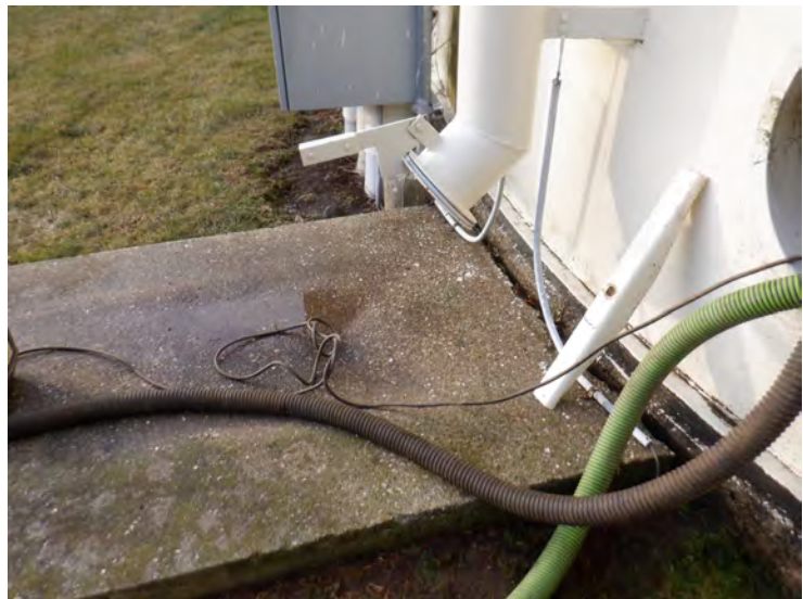
5) The overflow pipe discharges to a concrete splash pad.
