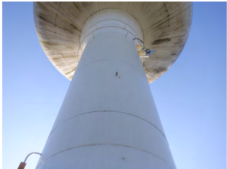
8) The riser coating is in good condition with no deterioration.
