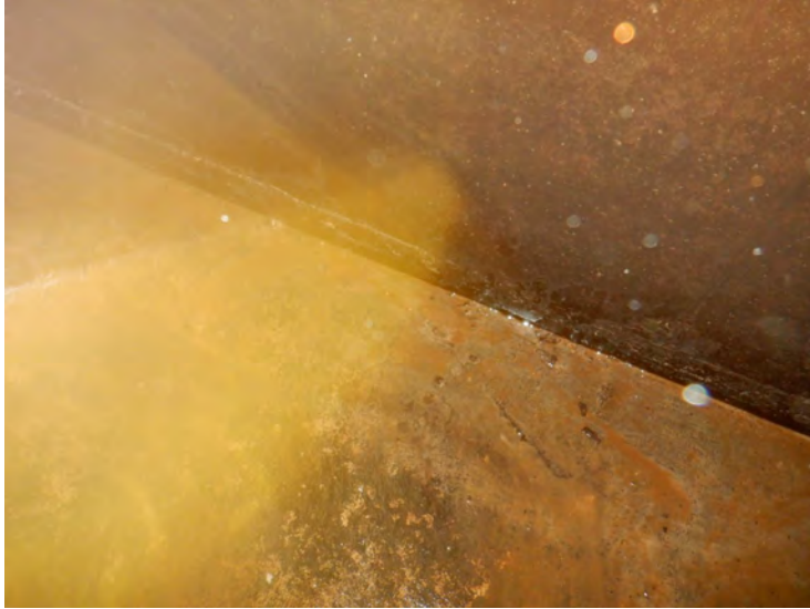
16) The wall to floor joint is in good condition.
