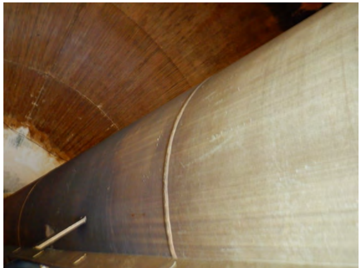
56) There are no coating failures on the access tube in the wet interior.
