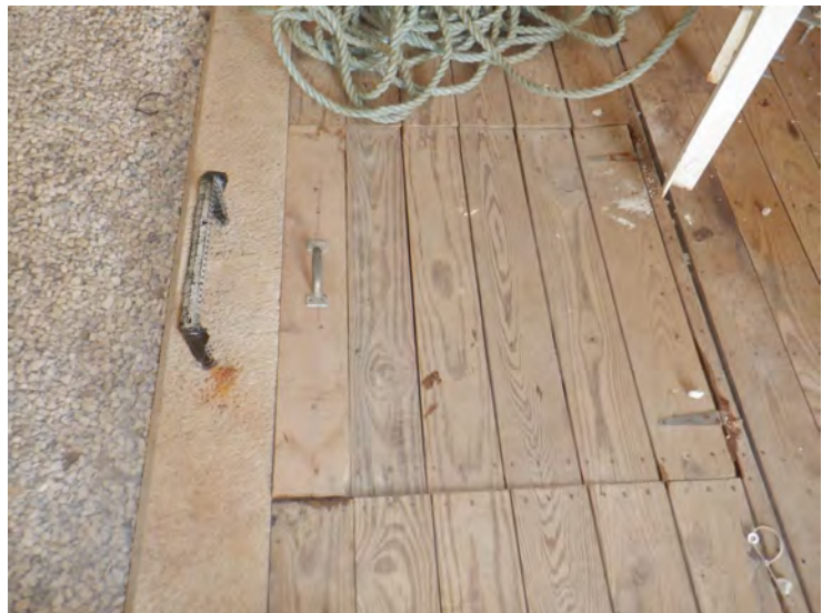
65) The wooden cover on the pit is in good condition.
