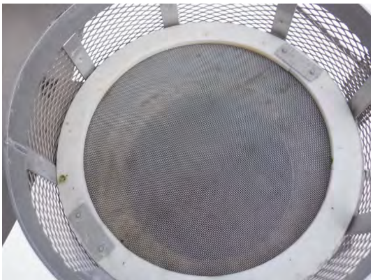
36) The interior screen is in good condition.
