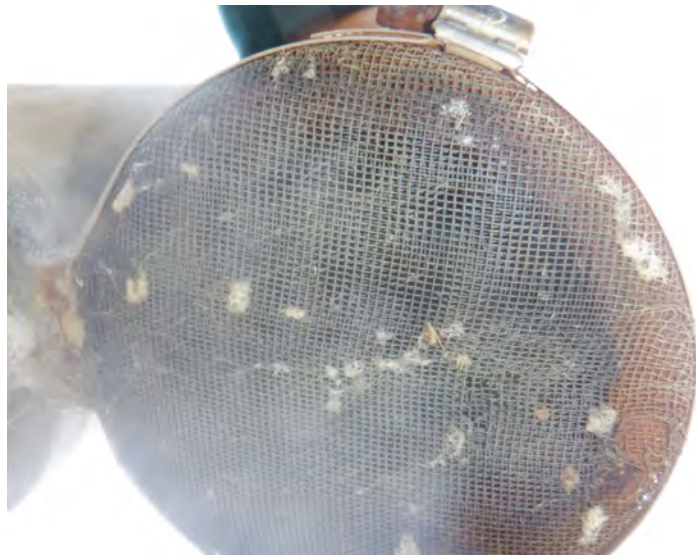
5) The roof vent screen is intact.
