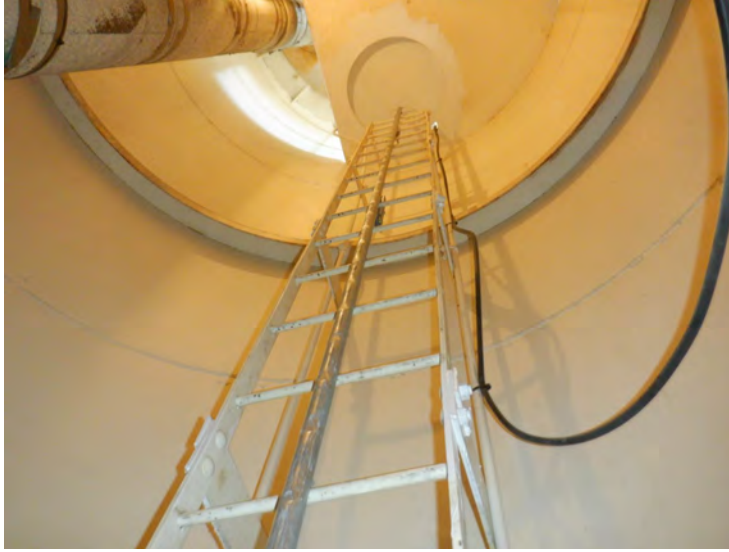
37) The riser ladder is in good condition. The ladder is equipped with a fall prevention device.
