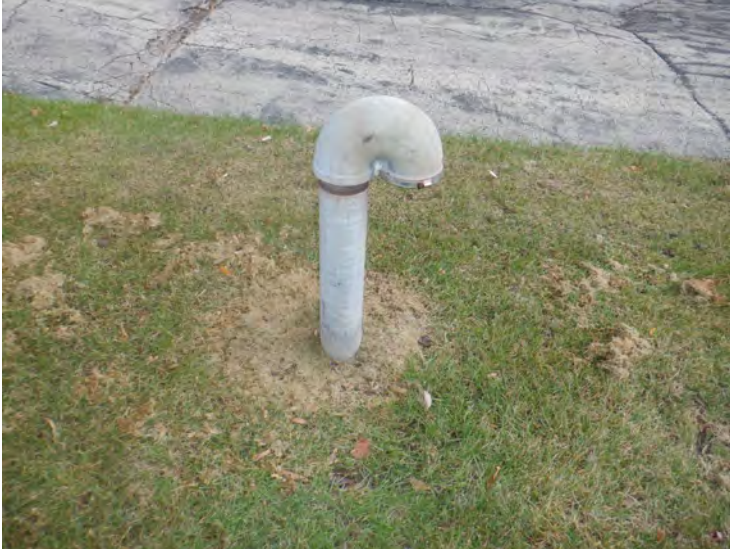
4) The goose neck roof vent is in good condition.
