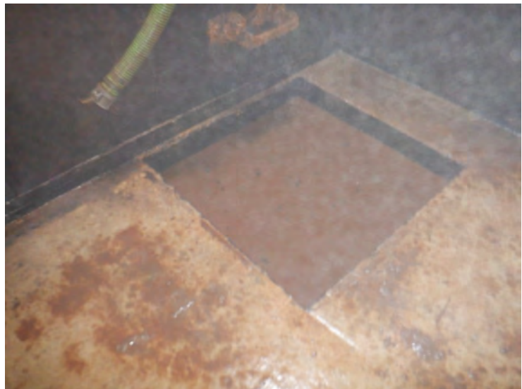
17) There is no deterioration of the concrete floor.
