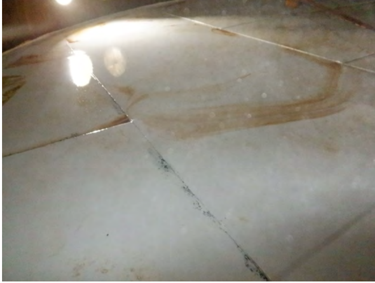
55) The coating on the floor is in good condition.
