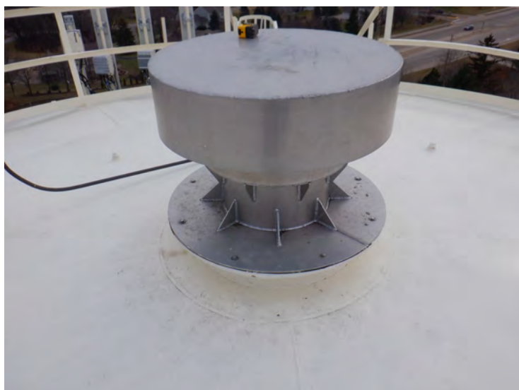
33) The roof vent is in good condition.
