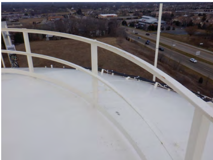
27) The center handrail is in good condition.
