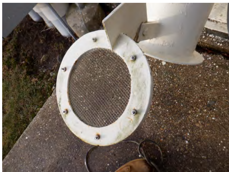
6) The screened flap gate is in good condition.
