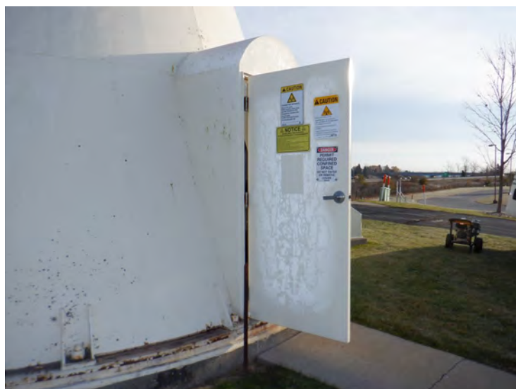
3) The service door operated properly during the inspection.
