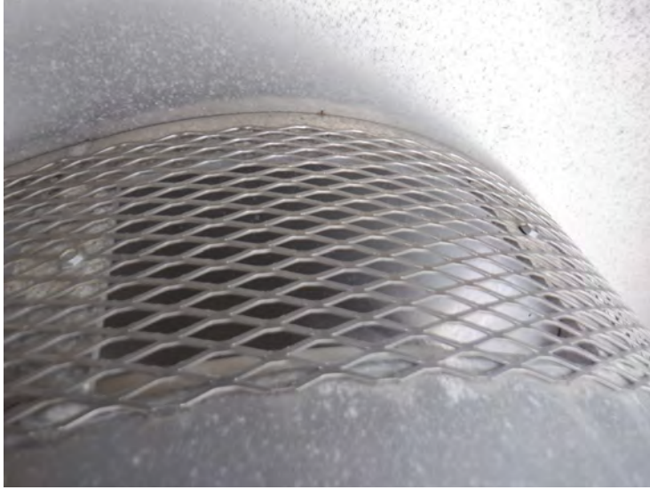
34) The vertical expanded metal screen is in good condition.
