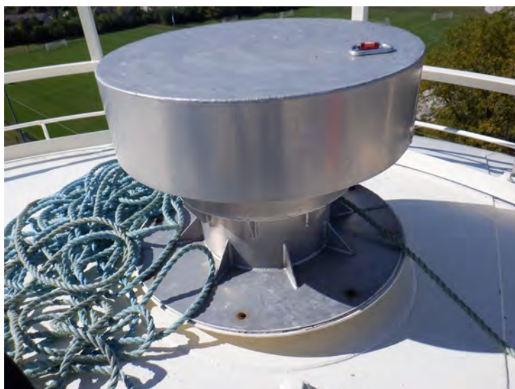
21) The roof vent is in good condition.
