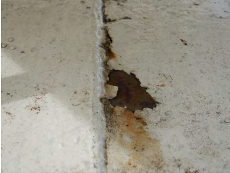
22) Spot coating failures on the roof.
