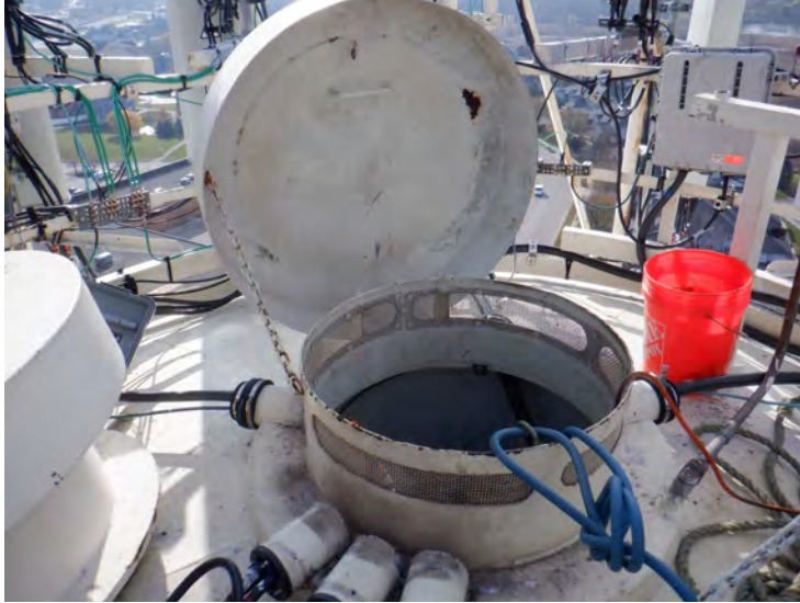
25) The dry interior roof hatch is in good condition.
