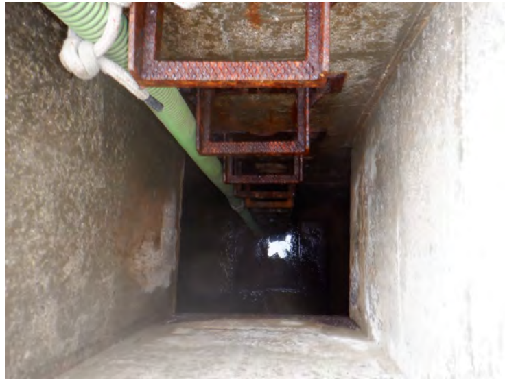
8) The ladder cleats from the roof to the floor are in good condition.
