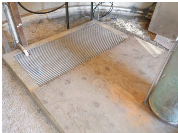
66) The cover over the pit in the basebell is in good condition.
