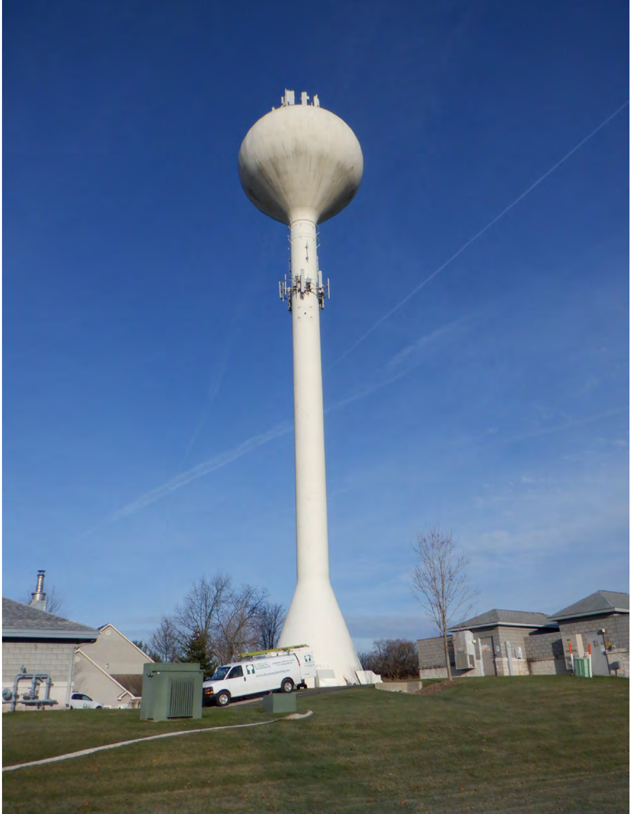
200,000 gallon spheroid (Quinlan Drive) elevated water storage tank owned by the Village of Pewaukee, Wisconsin.
