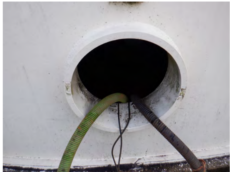
8) The two sidewall manways are in good condition.
