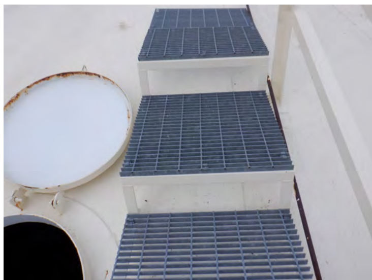
24) The steps to the center of the roof are in good condition.
