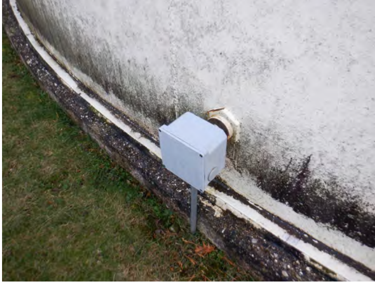
4) The cathodic protection pressure fitting is in good condition.
