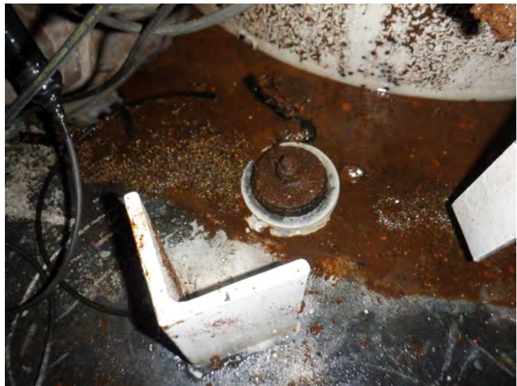
65) The mud valve operated properly during the inspection.
