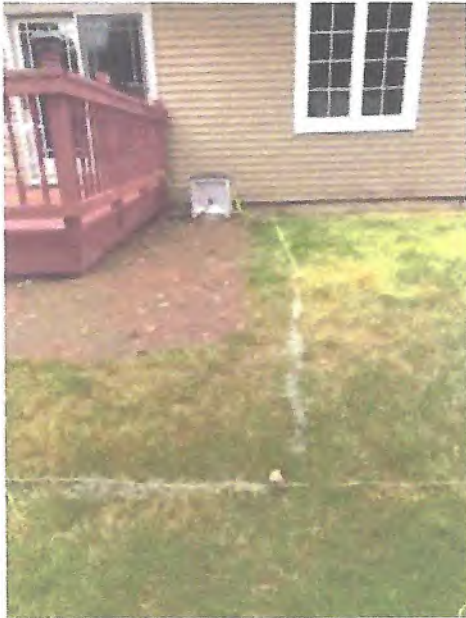
White Expansion Line on the South Side of my house. The 2nd set of stairs Will be added to this side of the new deck
