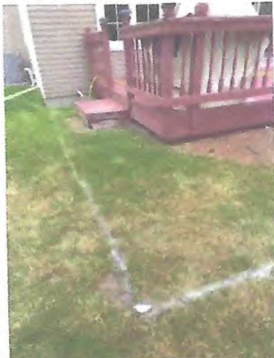
White Expansion Line from the side of the deck by the stairs
