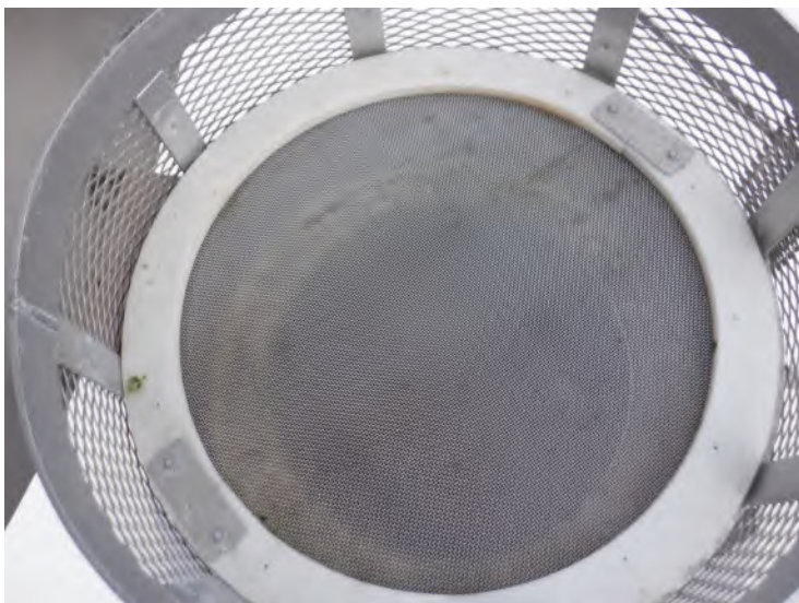
36) The interior screen is in good condition.
