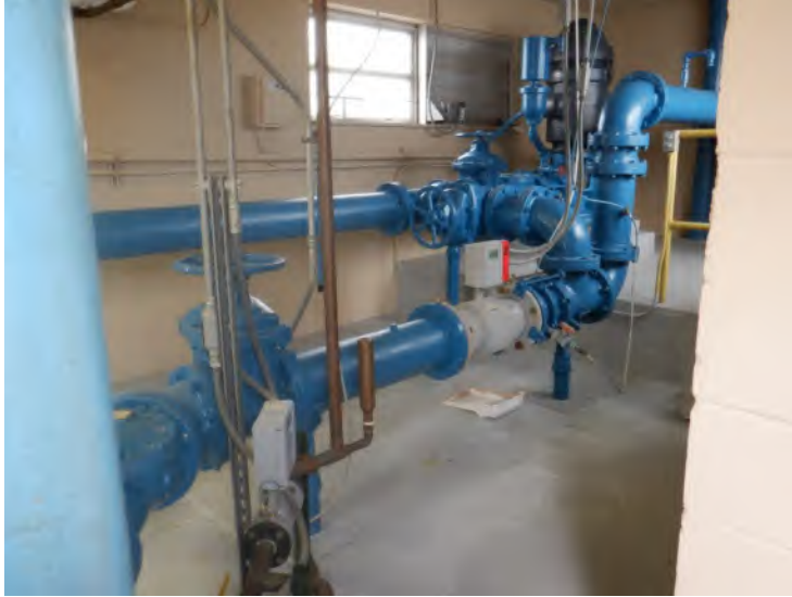
19) Coating on the piping in the pumphouse is in good condition overall.
