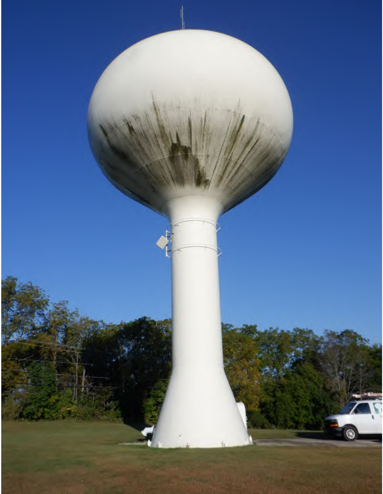
250,000 gallon spheroid (Lake Street) elevated water storage tank owned by the Village of Pewaukee, Wisconsin.
