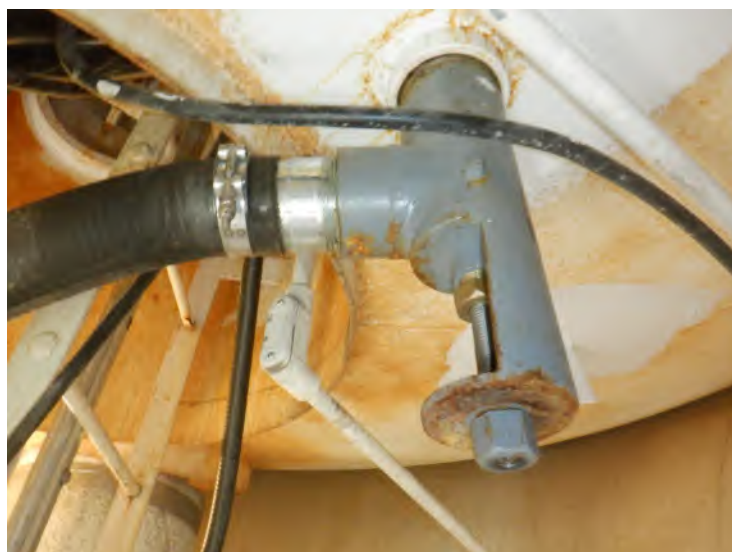
42) The mud valve operated properly during the inspection.
