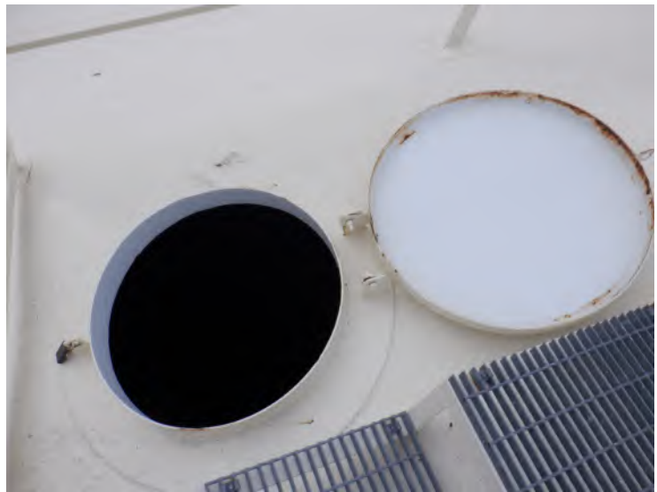
38) The roof hatch is in good condition.
