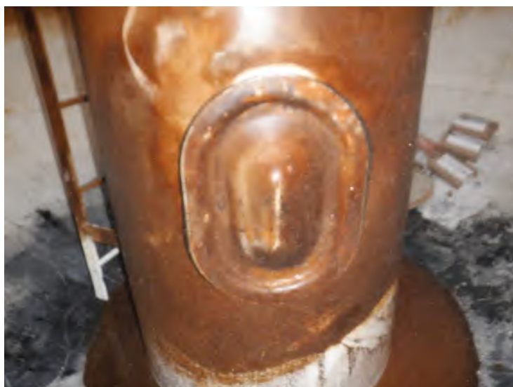
60) The wet interior manway cover is in good condition.
