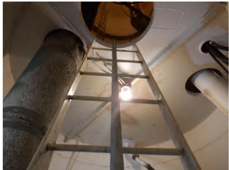
29) The baseball ladder is in good condition. The ladder is equipped with a fall prevention device.
