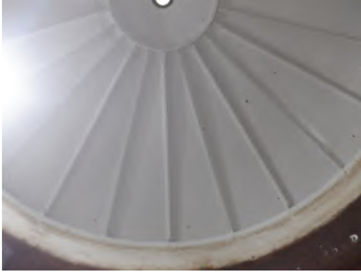
40) The coating on the roof is in good condition overall.
