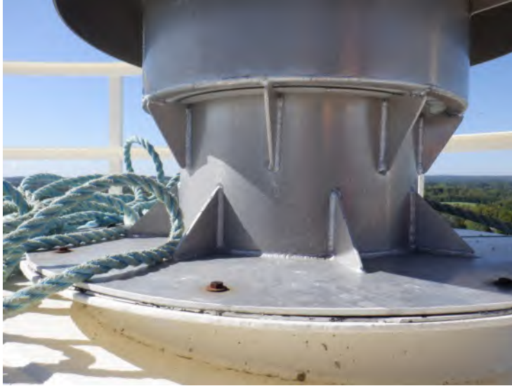
22) The roof vent pressure plate was properly aligned and free to move.
