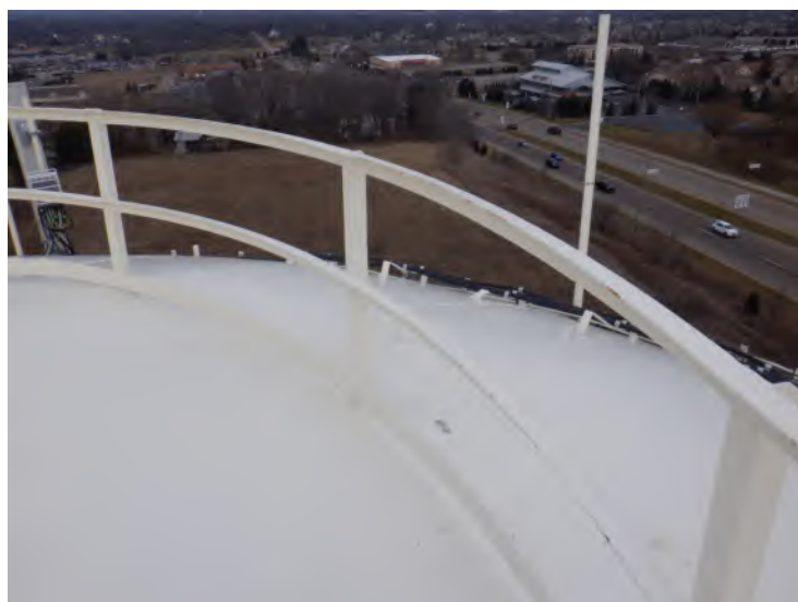
27) The center handrail is in good condition.
