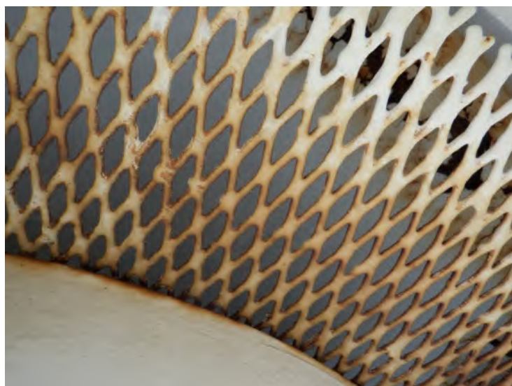
27) The roof vent screen is intact with no gaps.
