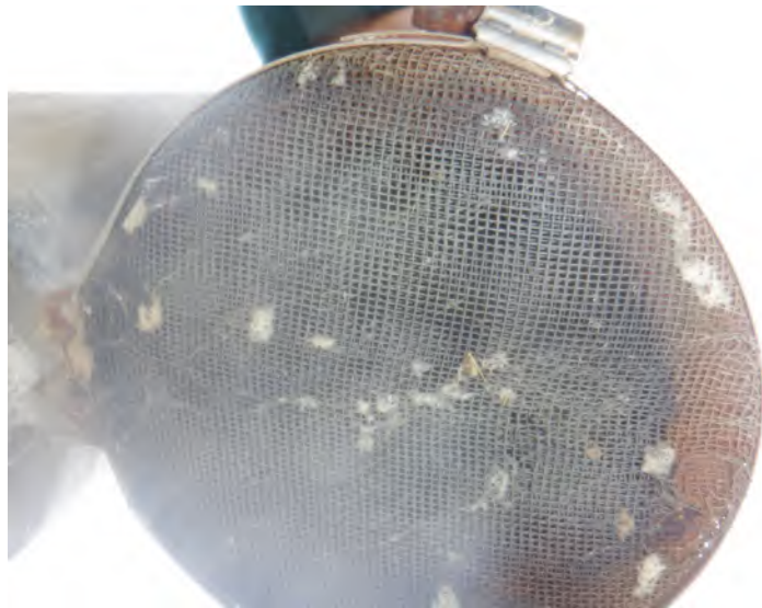
5) The roof vent screen is intact.
