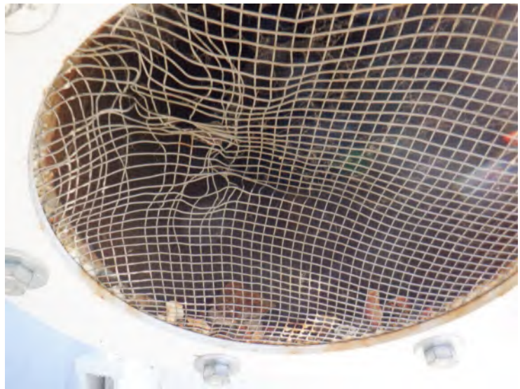
5) The screen at the overflow discharge is intact but deformed and oversized.
