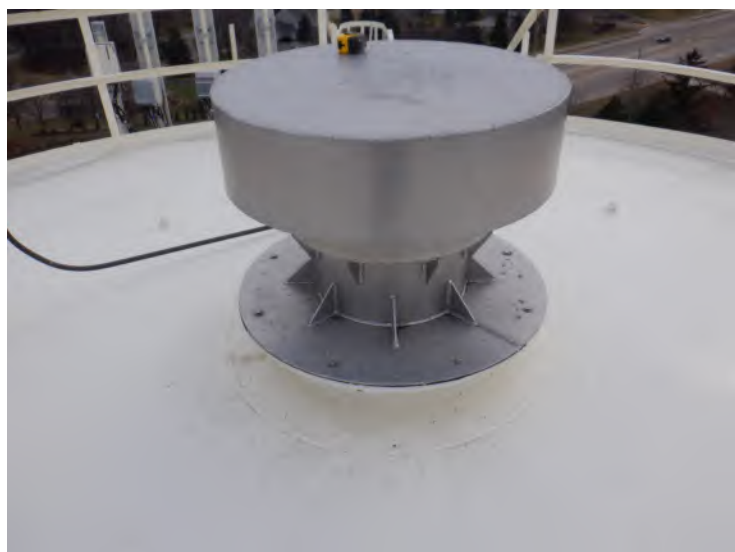
33) The roof vent is in good condition.
