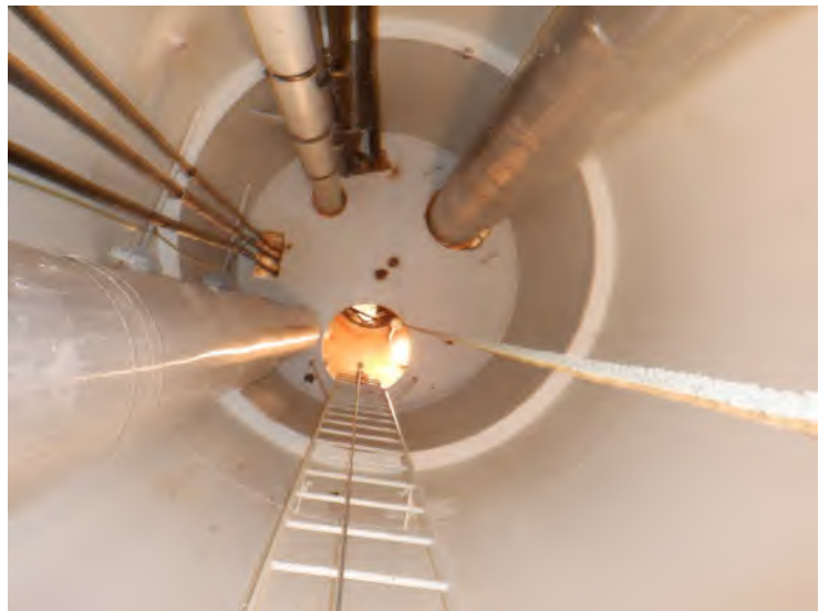
41) The riser ladder is in good condition. The ladder is equipped with a fall prevention device.
