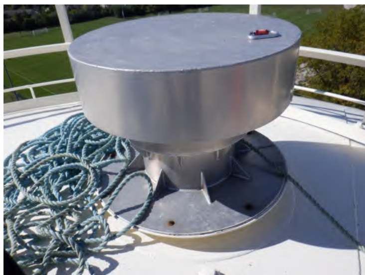
21) The roof vent is in good condition.
