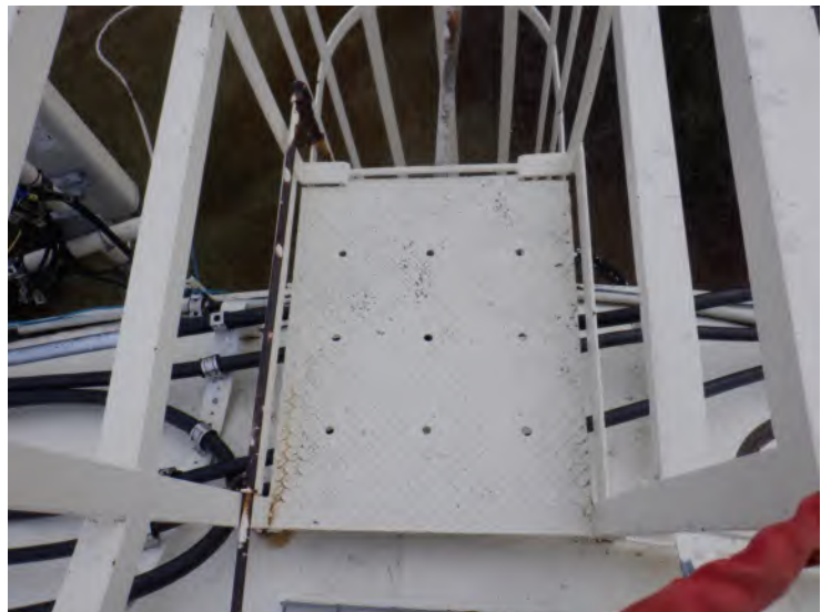
23) The step-off platform is in good condition.
