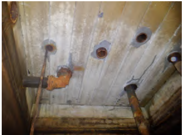
11) The fill pipe stubs at the wet interior roof.
