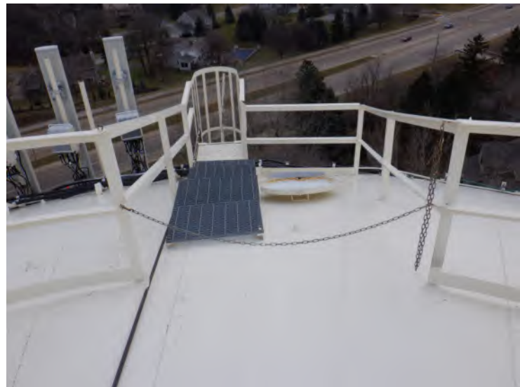
26) The step-off platform and roof hatch are surrounded by a handrail that is in good condition.
