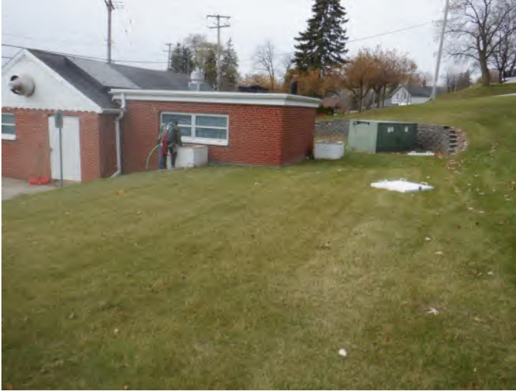
1) 125,000 gallon underground concrete water storage reservoir (Well 2) owned by the Village of Pewaukee, Wisconsin.
