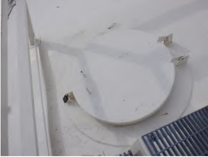
37) The roof hatch is secured with a padlock.
