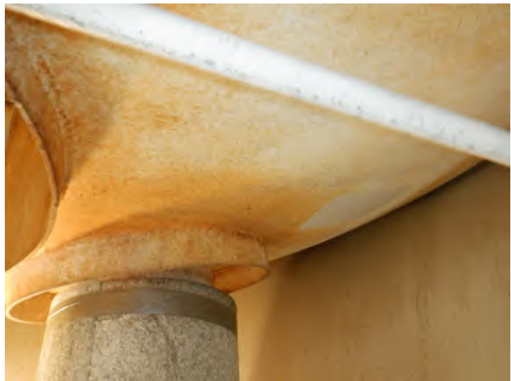
44) Extensive rust bleedthrough on the bowl.
