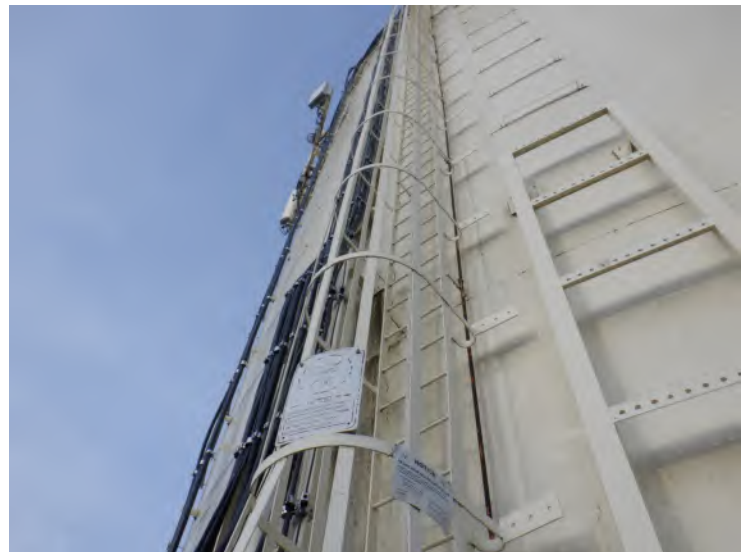
11) The sidewall ladder and cage are in good condition.
