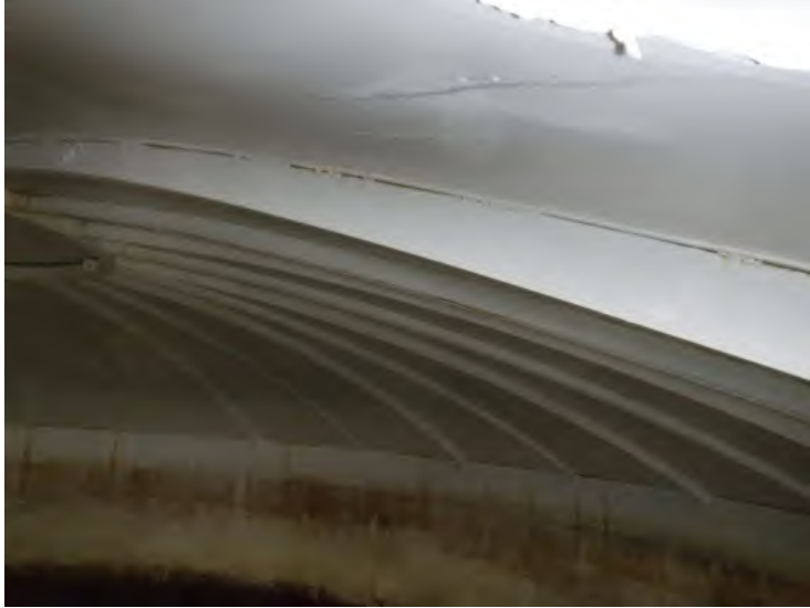
43) The roof stiffeners are in good condition.
