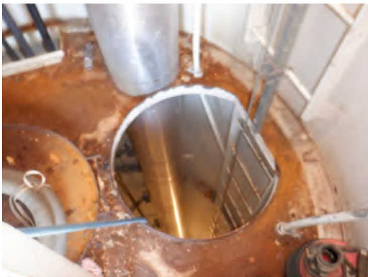
42) The ladder opening at the top platform is equipped with a hinged cover.
