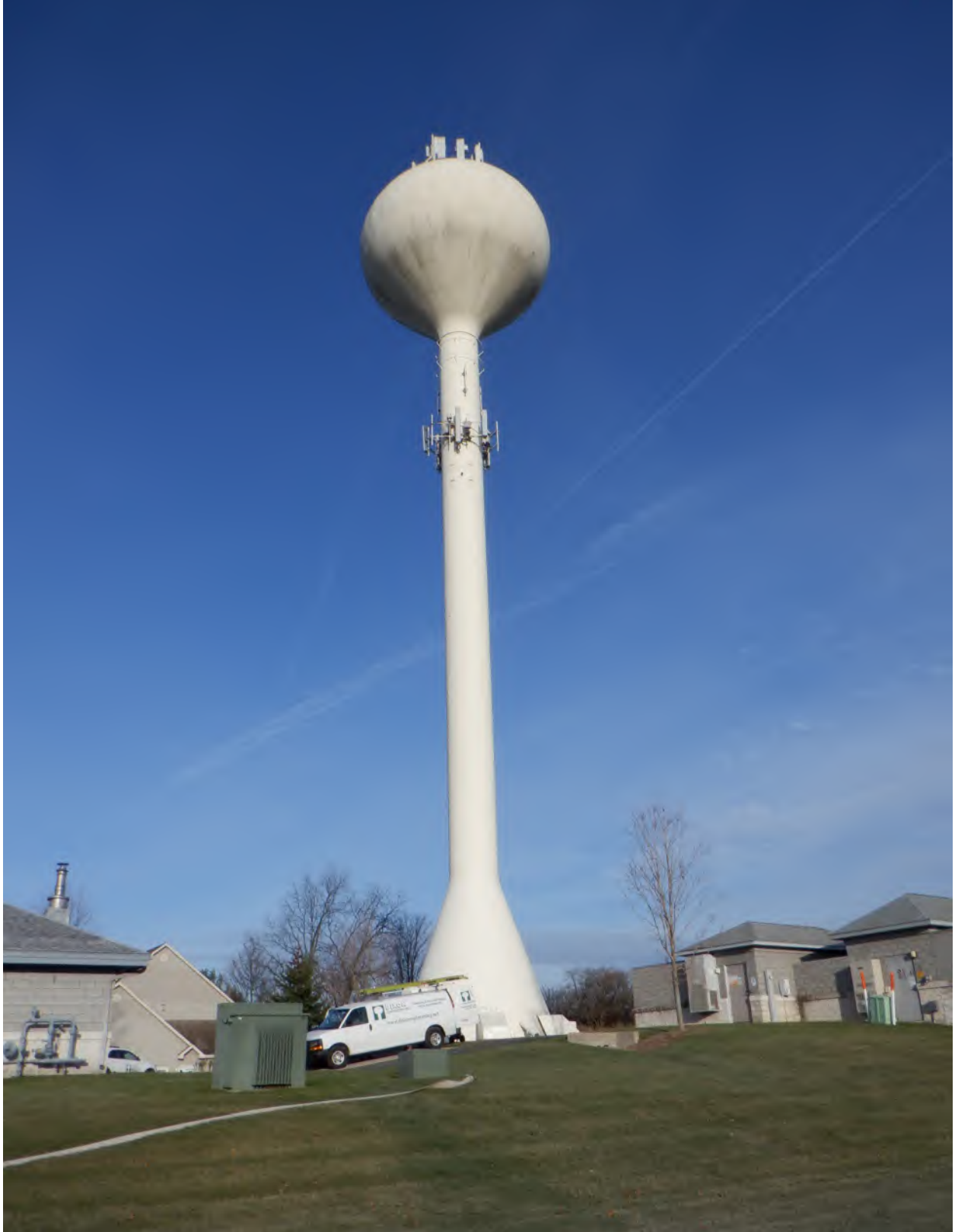
200,000 gallon spheroid (Quinlan Drive) elevated water storage tank owned by the Village of Pewaukee, Wisconsin.
