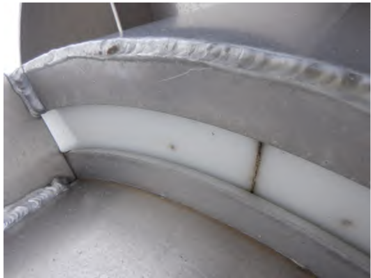
35) The pressure plate is in good condition.
