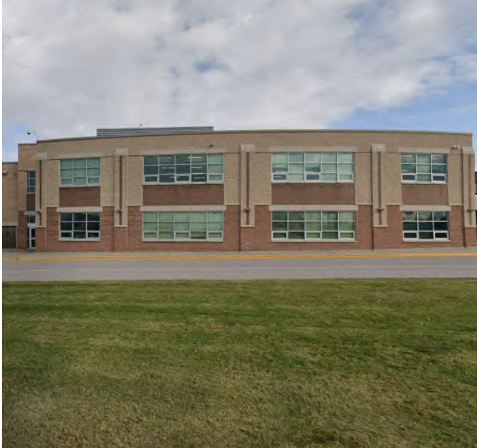
The older additions layer and alternate materials, creating a quilt-like articulation of materials.
