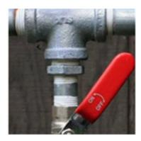
**Galvanized iron or steel.** If the pipe is silver or gray, hard to scratch with a key or coin you may have an iron or steel pipe. If you place a magnet on the pipe and it sticks to the pipe, you may have galvanized steel pipes.
